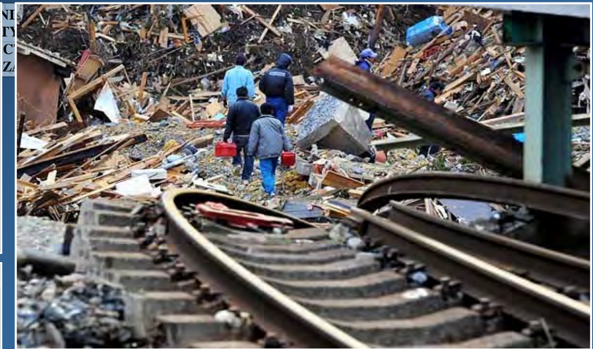
XII ITIS 2012 : Railway tracks damage, (NE JAPAN 2011).
