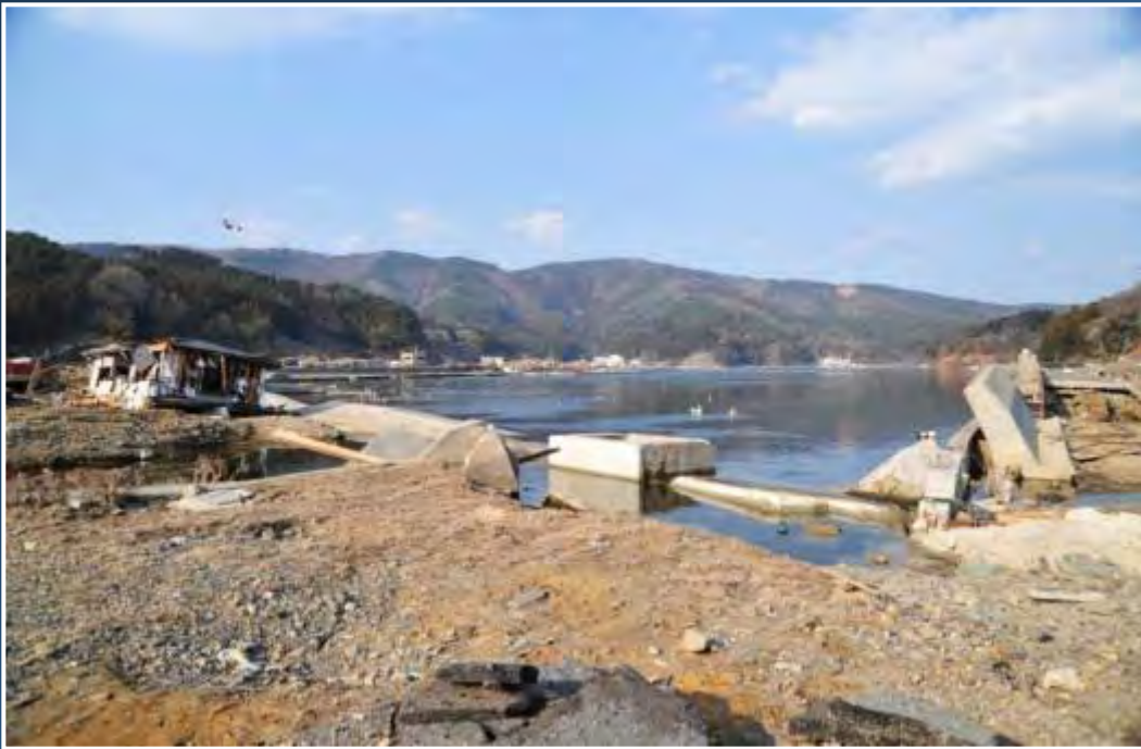
XII ITIS 2012 : Failure on antierrosional works on the shoreline.
