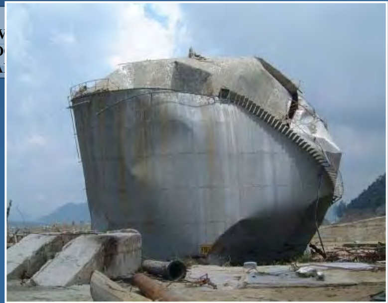
XII ITIS 2012 : Tanks on port facilities are moved
