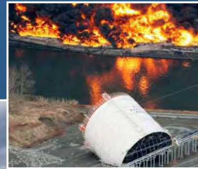
XII ITIS 2012 : Tanks on port facilities are moved
